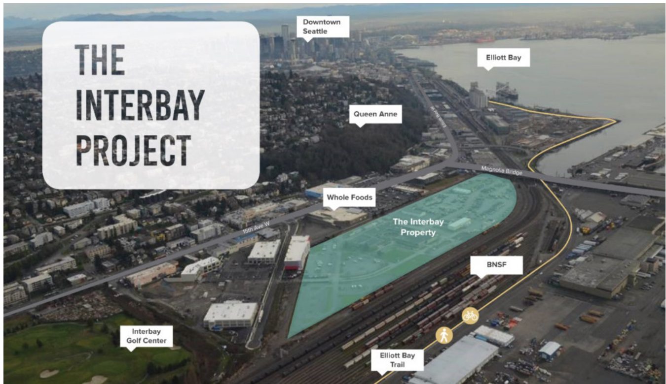
Figure 1. The Armory Site viewed from the northwest. Image credit. Washington State Department of Commerce.
